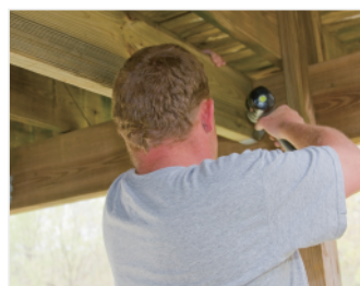
Wood structure repair
