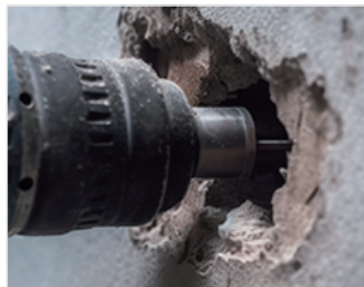
Curtain wall installation, stone dry-hanging skeleton fixation
