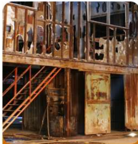
steel structure factory building
