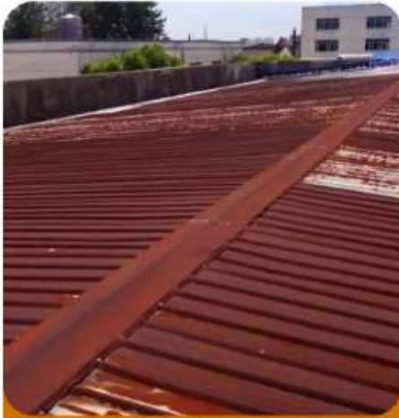
Color steel tile refurbishment
