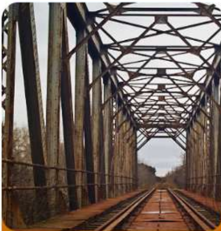
Steel structure bridge
