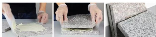
Glue with a plastic scraper
