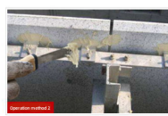
4-2: Apply the blended glue to the bonding surface
