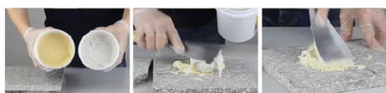
Remove AB glue with a putty knife
